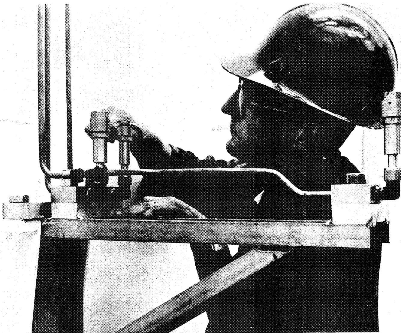
Fig. B-7 Typical installation of pressure transducers. Three transducers are shown attached to wall-mounted bracket. Lead wires exit through steel tubing.
