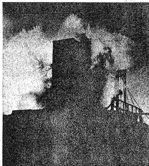
FIG. 7. Borax-1 shutting itself down safely by water expulsion after being made supercritical by 2.1%  $k_{eff}$
