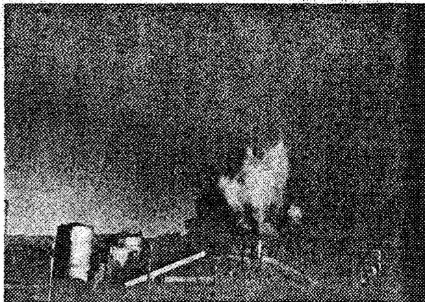
FIG. 8. When a 4%  $k_{eff}$  control rod was 80% ejected from Borax-1's core there was a light flash as reactor power peaked near  $1.9 \times 10^{10}$  watts, then a dark gray column appeared
