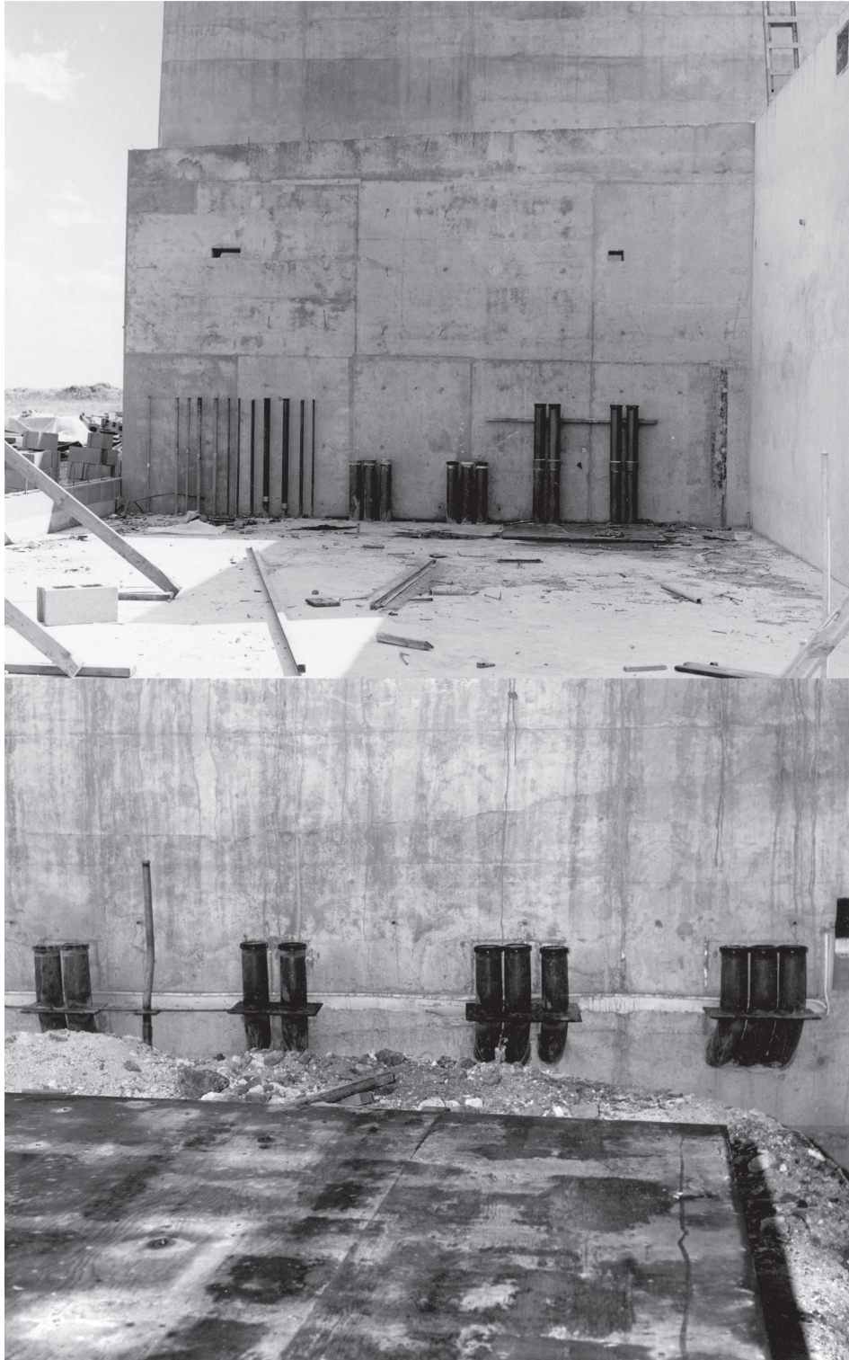
Fig. 12. Conduit along the south wall of the Control Room (top) eventually carried electrical and electronic cables into the Assembly Room (bottom) and the rest of the Hot Area. The two sets of three and two sets of two large-diameter conduits in the Control Room (top) in this August 31st photograph match up with the same conduits along the north wall of the Assembly Room (bottom) in this July 23rd photograph. The top photograph is looking south; the bottom, north.
