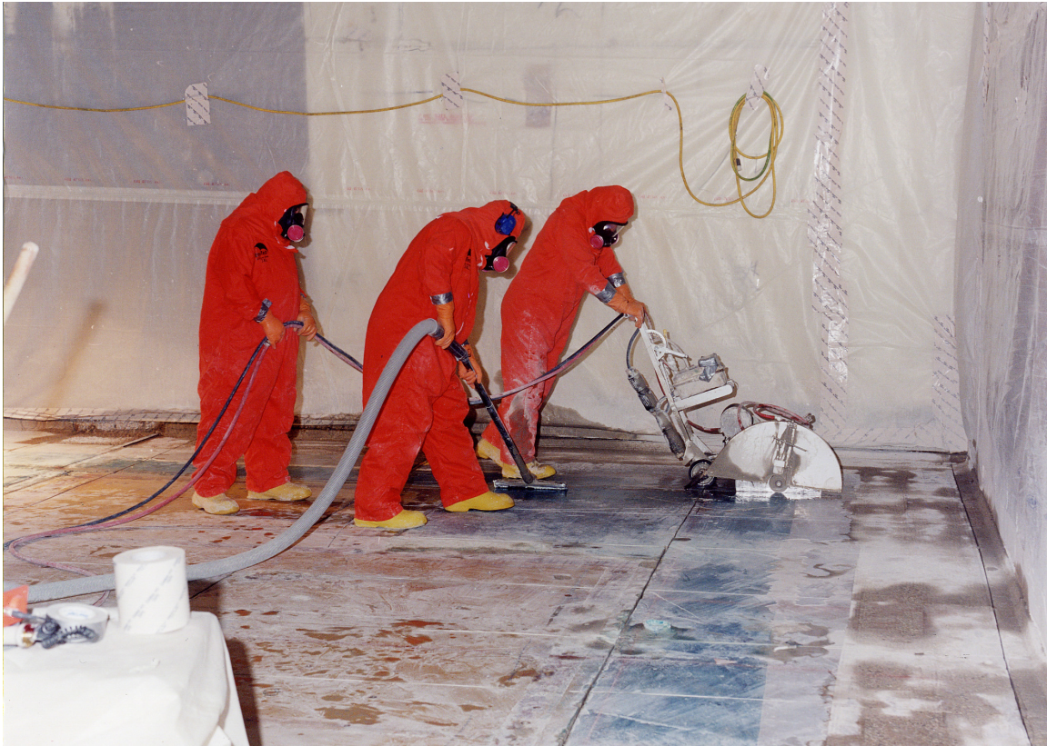
Fig. 85. The floor of the Assembly Room was sawed into rectangular chunks and lifted using the Building's 5-ton crane. Workers and the environment had to be protected from possible low levels of radioactive contamination. This scene was dated March 4, 2002.
