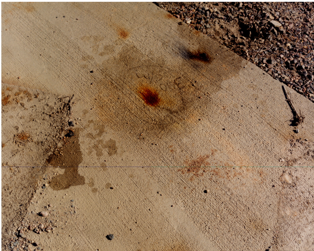
Fig. 134. The outdoor concrete platform which had supported the Portable Liquid Dumpster tank for decades was discovered to have very low uranium contamination on it. This discovery happened September 26, 1989. The tank's contents had been discharged into an open pond for evaporation for a few years; but the tank had been out of service for the previous 15 years. Atmospheric condensation inside the tank eventually leaked through decaying valve flange gaskets causing the incident.
