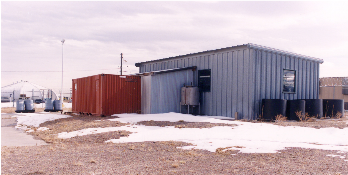
Fig. 81. The Storage Shed was a simple sheet metal building built upon a concrete slab. The commercial Cargo Carrier to the building's left was displaced a few meters to permit construction of a two-sided enclosure to produce a little additional storage area. Still, many items were simply left out in the weather. The four black objects against the west wall of the Shed (right) were neutron reflector/moderator pieces associated with the Shielded Annular Tank program. The nearly square, H=D , stainless steel tank (center) had been used for a number of non-fissile experiments involving Raschig rings. That important study investigated the size of void spaces within a bed of rings which might go undetected during a standard plant volume-calibration of such a tank. The surprising result of this study was that a critically large volume could escape detection unless careful scrutiny of the calibration data was performed. The grey drums in the background stored boron-rich earthen materials often used in casting plaster or concrete components for nuclear experiments. (February 1994)
