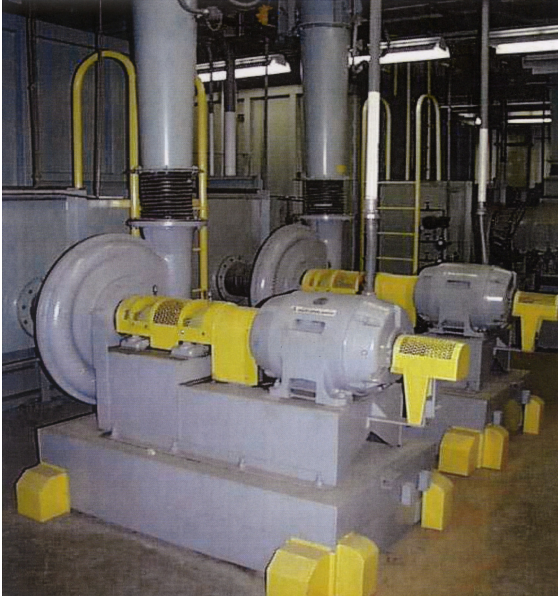
Fig. 78. Two blower motors provided suction on each portion of the building (Cold Area and Hot Area) through each filter plenum (Fp-501 and FP-502); but they were used in alternation. One was operating while the other was idle.
