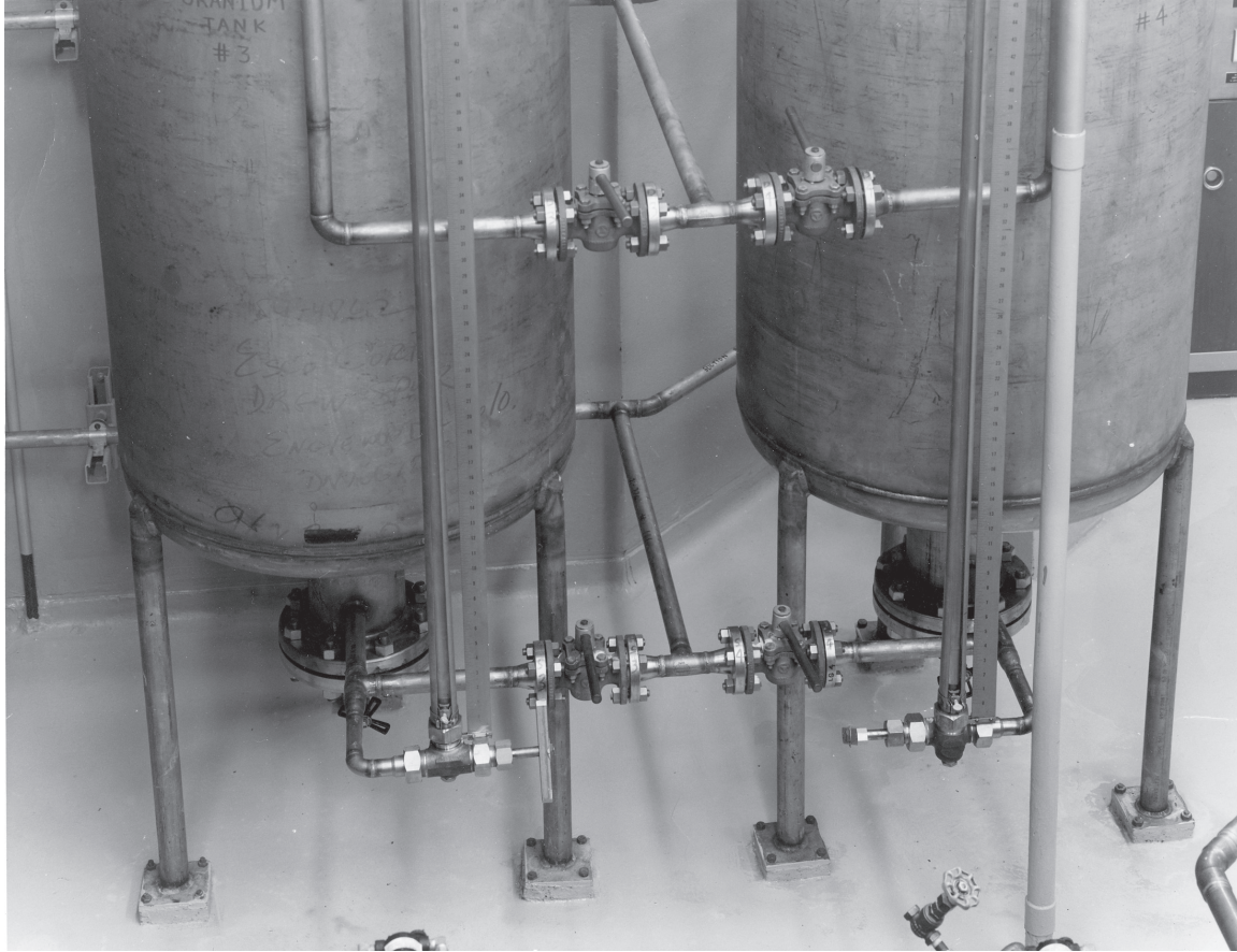
Fig. 44. Tanks were filled through the header at the top of the photograph and drained via the header near the bottom. Other details, such as Sight Gauge and valving, are discussed in the text and clearly illustrated here. (May 1965)
