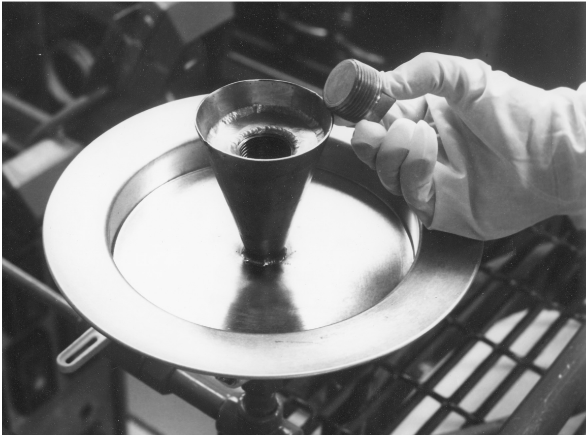
Fig. 54. Small quantities of uranium solution were re-introduced into the tank farm through this funnel assembly located above the tanks and on the Line Drainage Distribution Header. The screwed plug precluded dirt and dust; and the drip pan prevented contamination of the floor far below.
