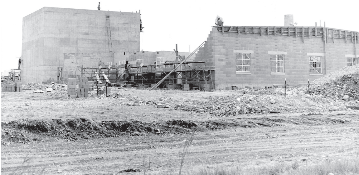
Fig. 11. The walls of the office area had just been started by August 20, 1964, (top); but 11 days later, the north wall (bottom) was essentially finished. Cinder block along exterior walls and one interior north/south wall along the hallway was backfilled with rebar and mortar to provide load-bearing walls. The Assembly Room had been completed some time prior to August 20 since concrete forms are being removed in the top photo.
