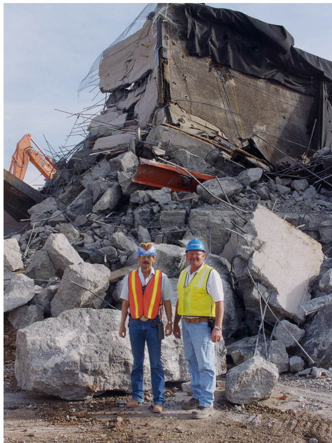
Fig. 90. The Assembly Room was reduced to a pile of rubble the day following explosive fracturing. James W. Smith and Richard Seago, associated with the demolition project, seem proud of their accomplishment that Sunday.
