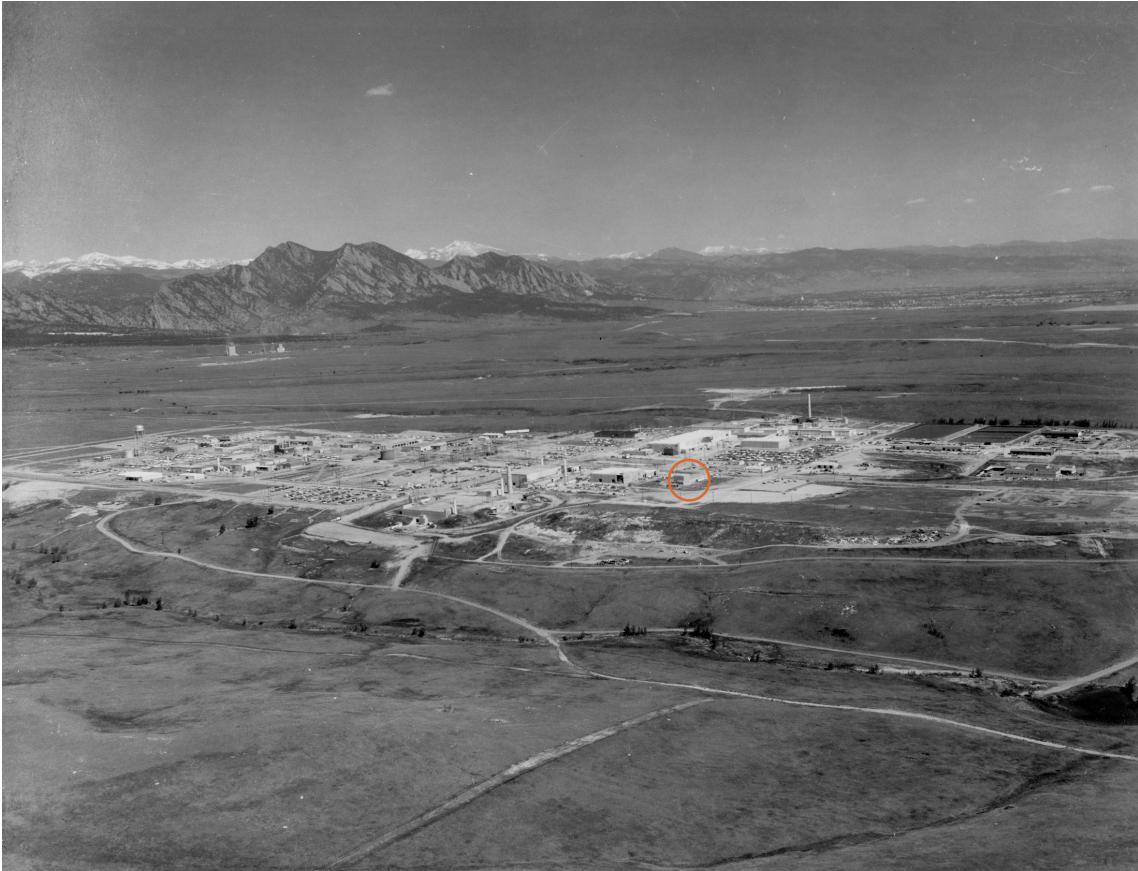
Fig. 1. An aerial view of the Rocky Flats Plant Site taken in June of 1969 shows the 5-year-old Building 86, now called Building 886, within the circle.
