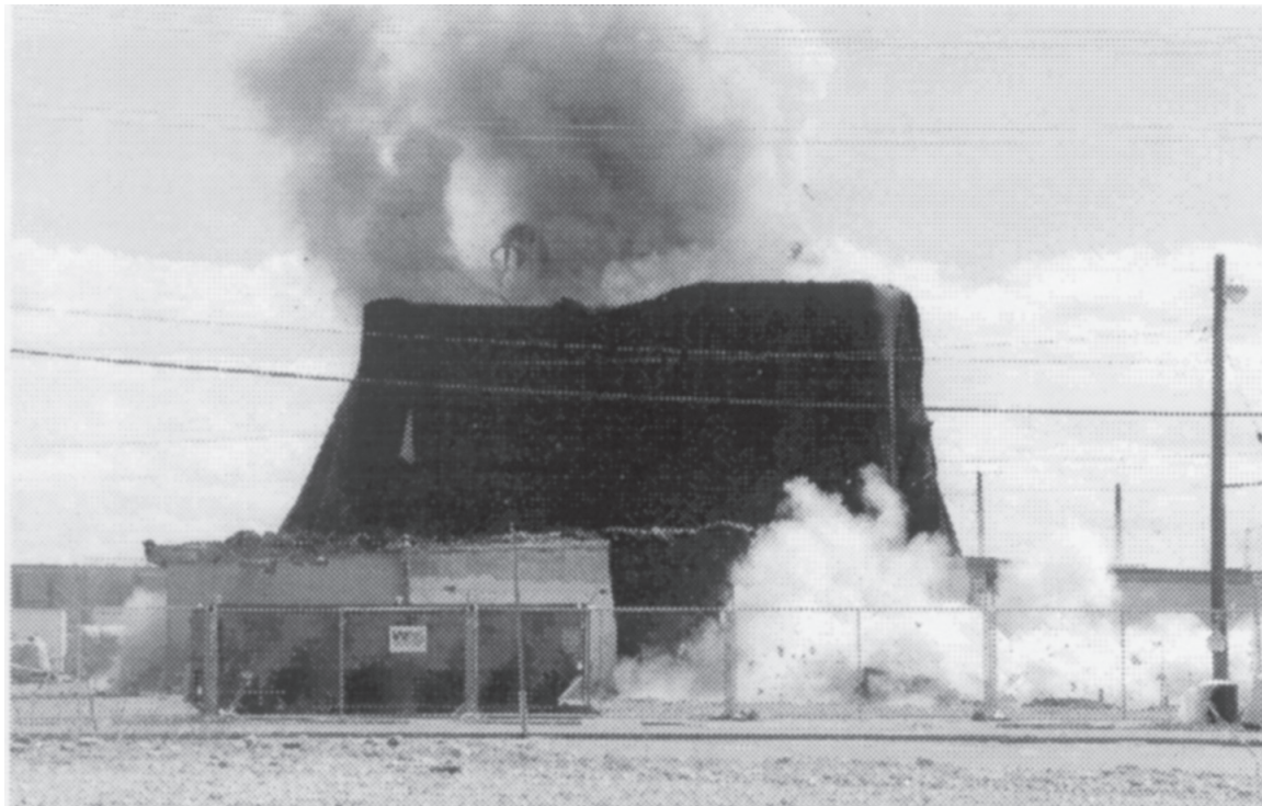
Fig. 88. The power of the explosion soon caused the shroud to billow away from the non-weakened Assembly Room as clouds of smoke and concrete dust tumbled into the air. The date was April 13, 2002.
