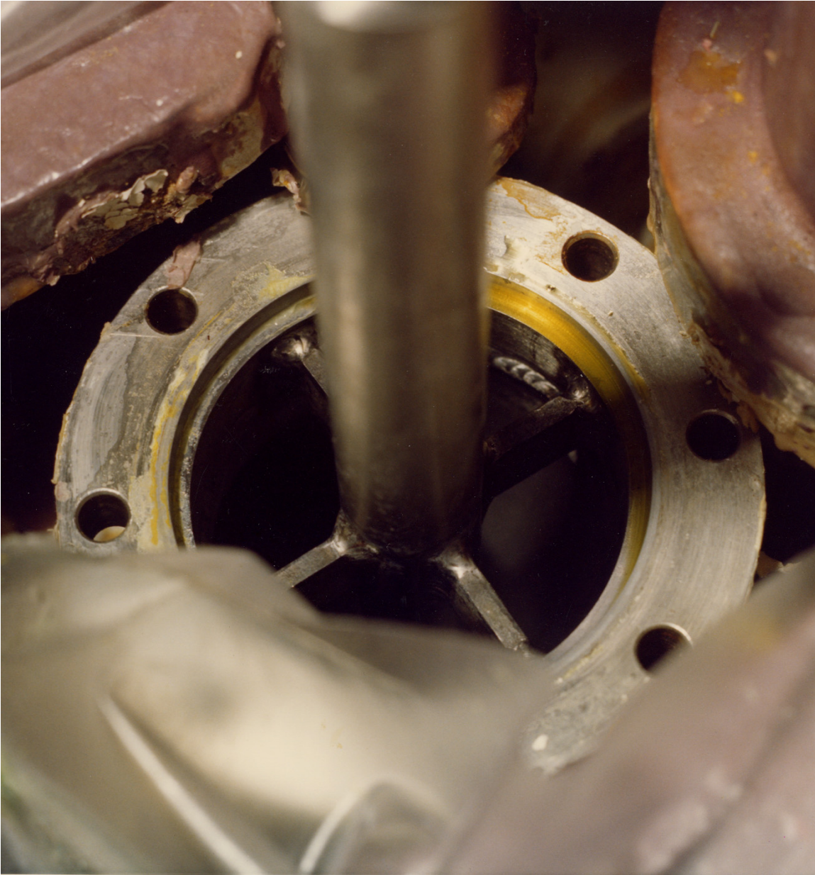
Fig. 26. The SCRAM valves were almost never disassembled; but this 1982 photograph shows the exception. The flanged joint is the mid-height of the valve. The centered guide tube for the operating plunger rises above the joint.
