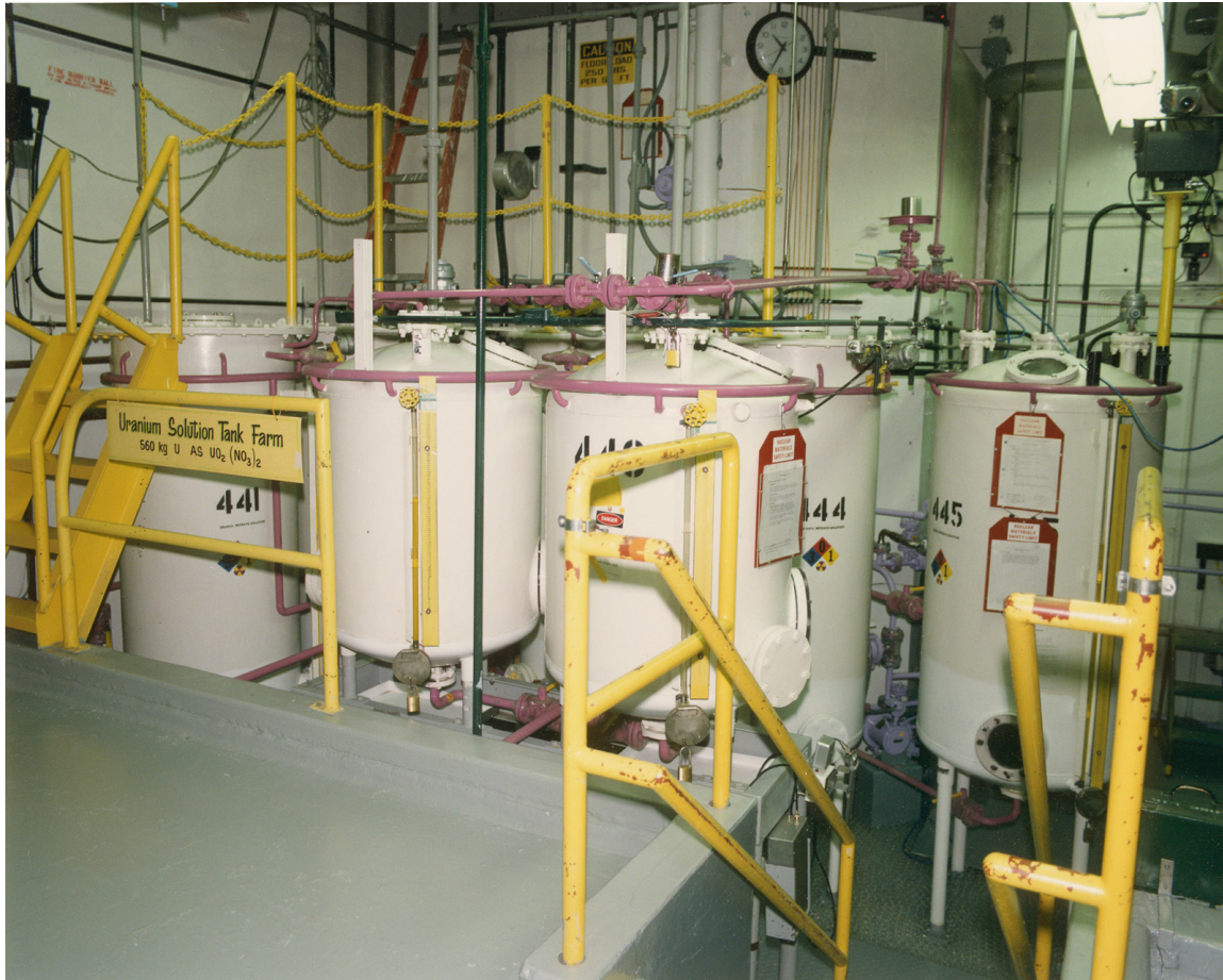
Fig. 59. No more experiments were ever performed at Rocky Flats after this photograph in July of 1990. Several of the final nine tanks are seen. Sight Gauges, spray rings, inspection ports, Criticality Safety limit holders, a large portion of the Line Drainage System (including the funnel input for small sample returns), the elevated manifold ventilating tanks, and the Tank Calibration Station (white vertical pipe to the left of the clock) are all shown. (July 1990)
