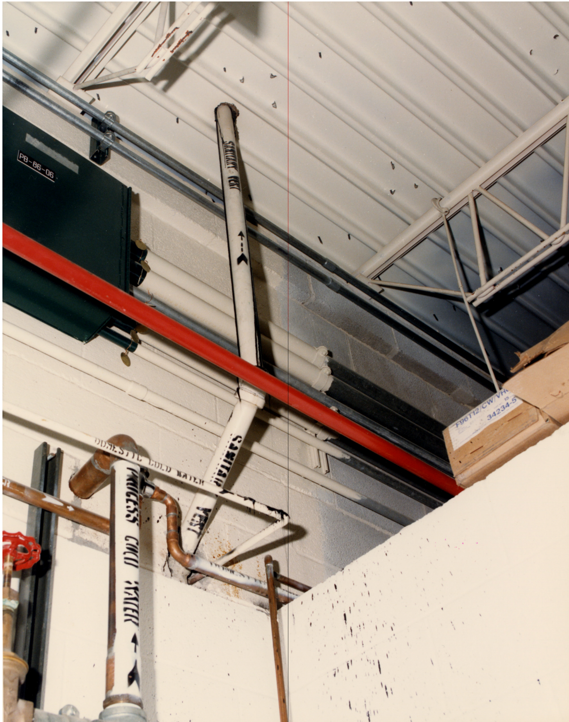
Fig. 132. Metal spikes driven through the metal pan roof formed the path for the tar to leak inside the building. The room shown is the janitor's closet.
