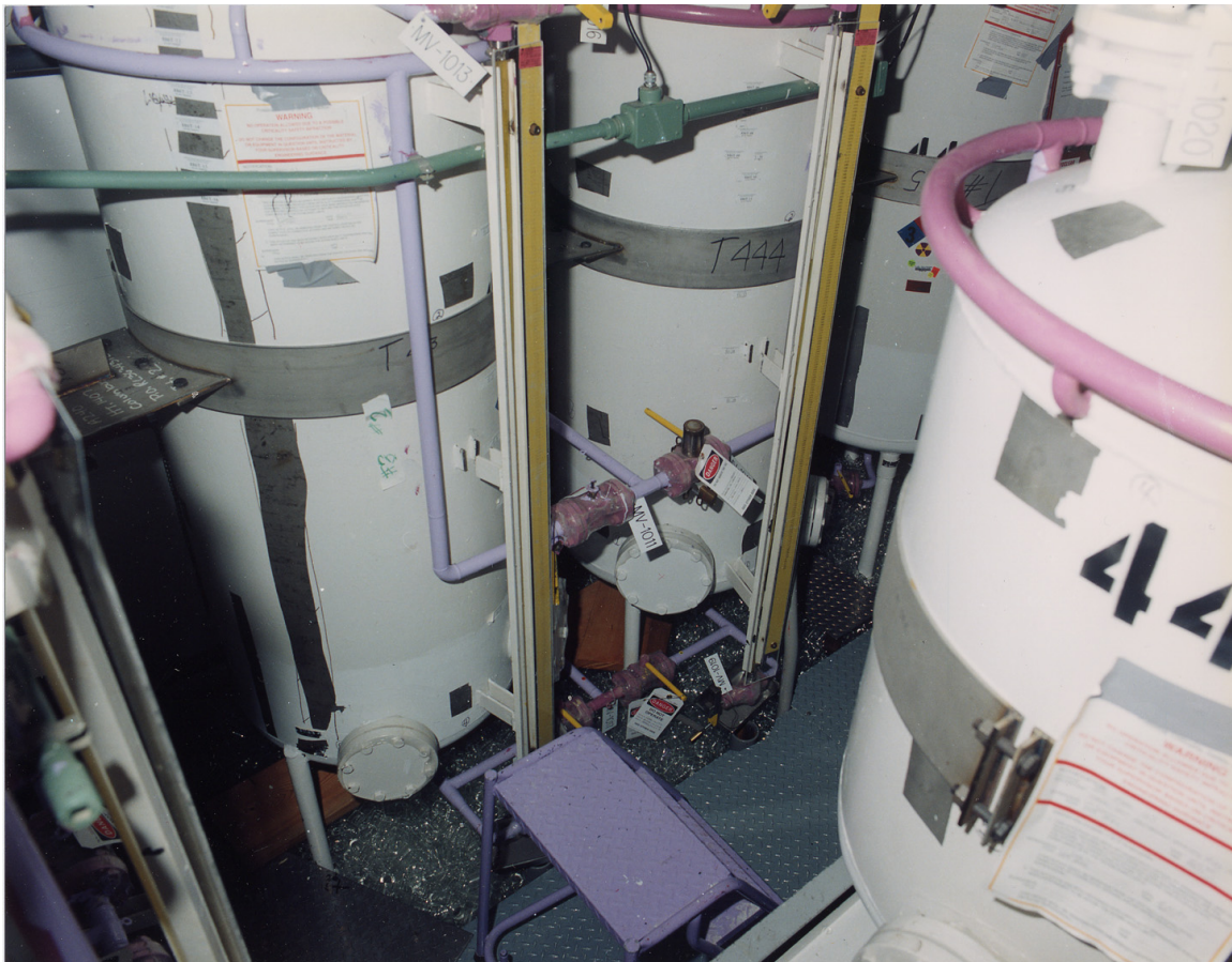
Fig. 64. All nine tanks were stabilized against seismic events while they still contained uranium solution but long after the useful life of the solution. Stainless steel “belly bands” were bolted to walls, in this April 1996 photograph.
