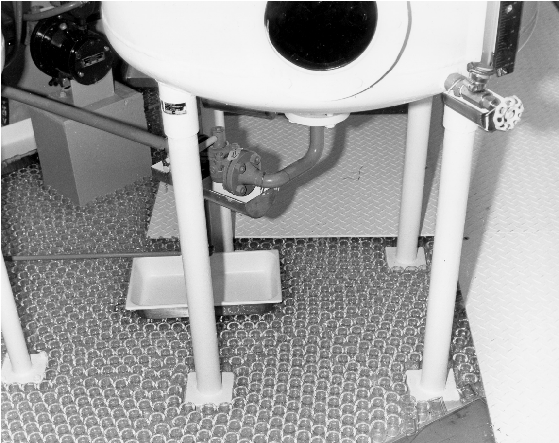
Fig. 63. The pit floor of room 103 was covered with a single layer of Raschig rings for about two decades, although the worth of this action is questioned. Metal boiler plate covered frequent walking areas in this March 1970 photograph.
