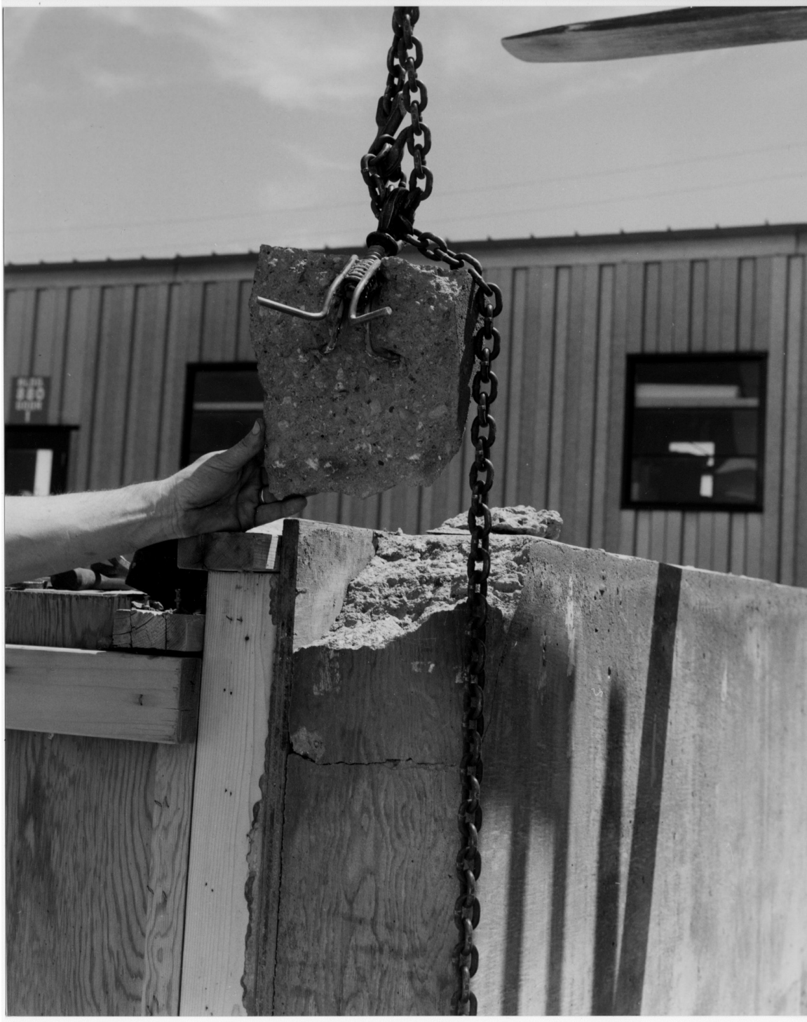
Fig. 119. This lifting anchor cast into a concrete wall section formed a weakened plane where four L-shaped rods fanned out. This break happened during manufacture before the wooden form could be removed.
