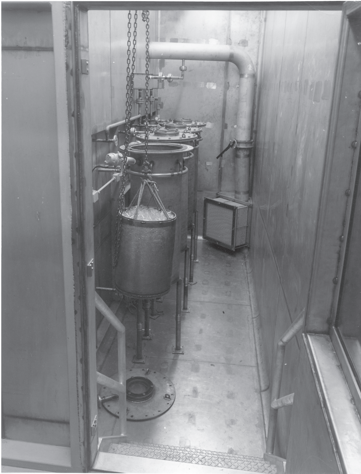
Fig. 45. The top basket of randomly oriented Raschig Rings are about to be added to the near tank in the stainless steel enclosure. These tanks were to have housed plutonium solutions; but that never happened. (May 1965)
