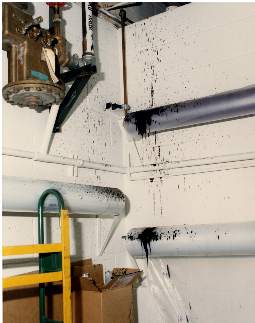
Fig. 131. Building 886 was almost 25 years and a new roof was to be installed. The old roof had never leaked but was removed to provide a fresh surface for a new tar-and-gravel composition. Fresh tar leaked through openings and damaged rooms inside the building. The janitor's closet had tar splattered onto walls and rolls of plastic sheeting.
