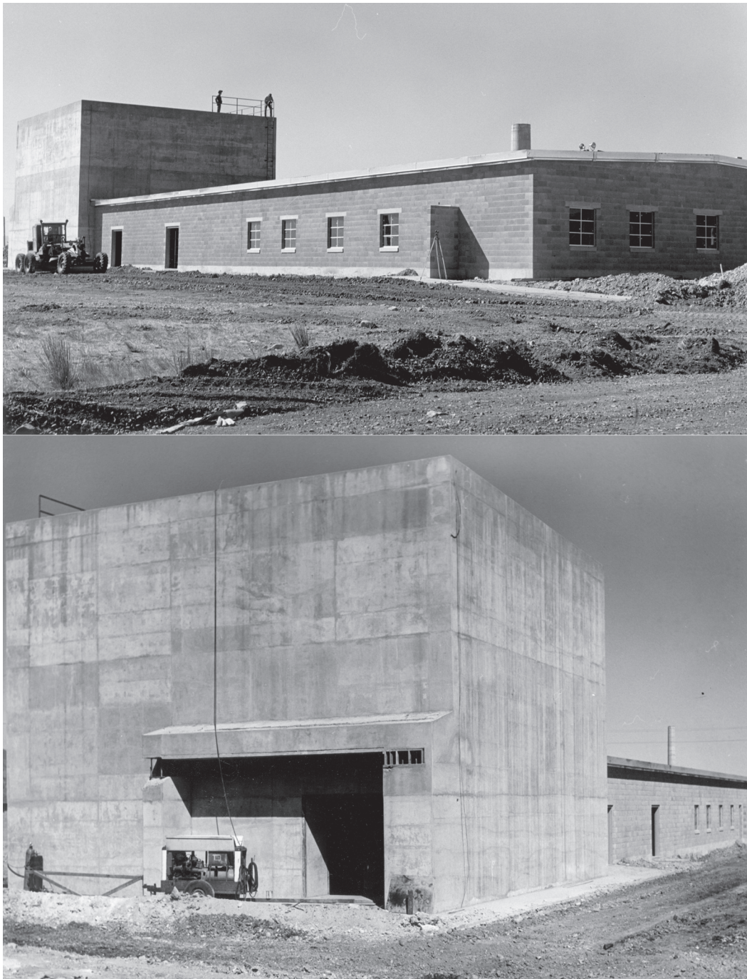
Fig. 15. The entire Building 86 appears nearly finished in this October 24, 1964, photograph (top). The view is looking southwest with the east wall bathed in sunlight. Two light-weight steel doors have not yet been installed. The near one opened to the Control Room. The one next to the wheel of the road-grader led to the Storage Vault—interesting in light of more modern safeguards measures. This room would contain several hundred kilograms of enriched uranium and plutonium metal. The cinder block wing projecting from the wall near the north end of the building was a shield against strong Colorado winds protecting the would-be main entrance to the office area. The bottom photograph was taken the same day and looks north and a little west. The heavy, thick, concrete Shield Door will be installed in the concrete projection off the south wall.
