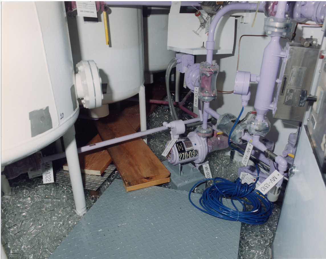
Fig. 62. Several aspects of the handling system discussed over several pages are illustrated in this 1996 photograph. The level of Raschig rings on the floor, greater than the single layer that had existed for decades, is that established during worries over seismic stability. Uranium solution was delivered to experiments at a high rate early during experiments and moved among tanks within the Mixing Room via the centrifugal pump just to the right of center (with the numbers '270-09' stenciled on its side). The Solution Sampling Port (top) consisted of two manual valves in series. One (not seen) was a simple on/off valve; and the second could throttle solution as slow as a drop at a time. The tubing nozzle has a "T-shaped" wire inserted up its snout to prevent salt crystals from hardening. A white-faced drip pan with two sides protects the floor from contamination. The Densitometer shows at the right; and the absence of a manual valve at the output of the FAST pump is noted. Labels and cables are associated with decommissioning.
