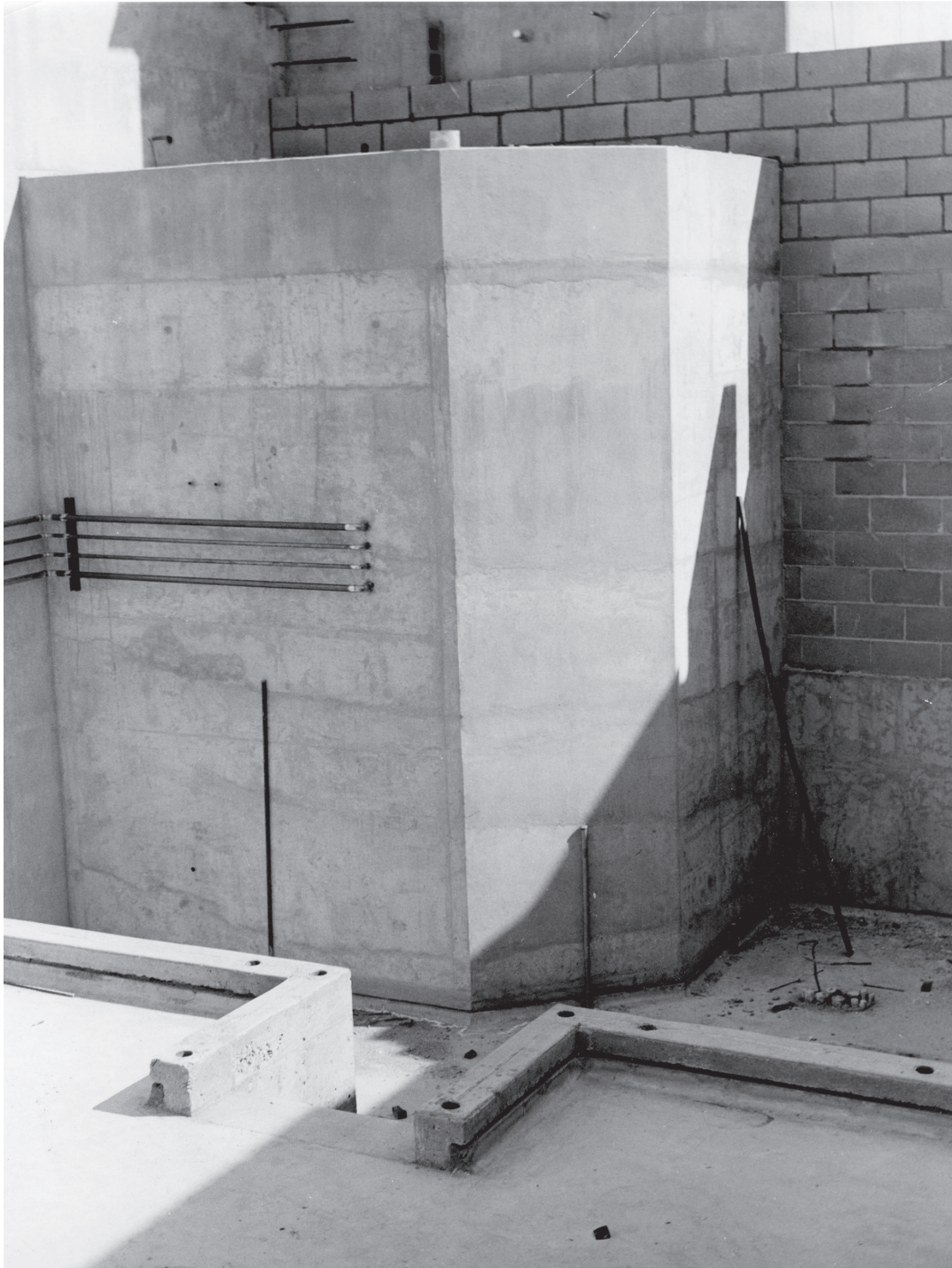
Fig. 14. Shadows grow on the Labyrinth wall in the depressed pit area of the Mixing room in this August 31, 1964, photograph. The notch in the upper level (foreground) will have steps to the Pit Area which later will house the Tank Farm.
