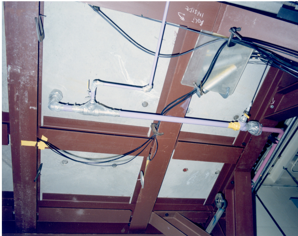
Fig. 20. The concrete Elevated Platform consisted of eight panels supported by a steel superstructure, supported, in turn, by steel legs. All of this except the poured concrete was made of structural steel shapes. A portion of one leg and diagonal bracing for two legs is seen at the right in this underside view of the Elevated Platform. Solution lines passed through holes precast into the slabs. Several radiation detectors can be seen connected to coaxial electrical cables.
