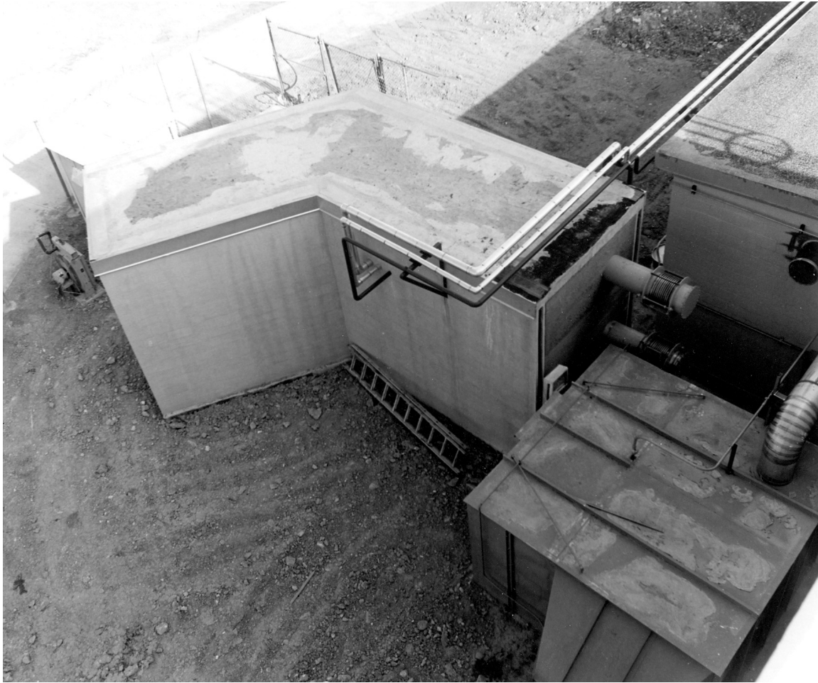
Fig. 79. The new Building 875 connected to the CML via an underground tunnel which rose above ground at the dogleg to the left of center. The above-grade portion has not yet been connected to Building 886. The top duct will bend and connect to the short penetration in the south wall of room 103. This will exhaust the Cold Area. The lower will connect to the duct (far right, below center) shown still connected to the original sheet metal plenum building. (May 1974)
