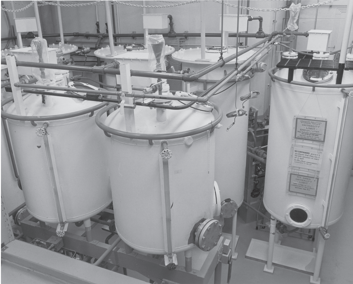
Fig. 49. The original four tanks (flat tops) were increased to seven by the addition of used tanks from another building by the time of this January 1969 photograph. The three are the rightmost and the two short tanks in the foreground. The view looks just east of straight south from the upper level into the pit area. Used tanks have dished tops as well as bottoms. Many features of the tanks are discussed in the text. Safety Limits posted on the tank to the right reveal the rather informal format permitted in 1969.
