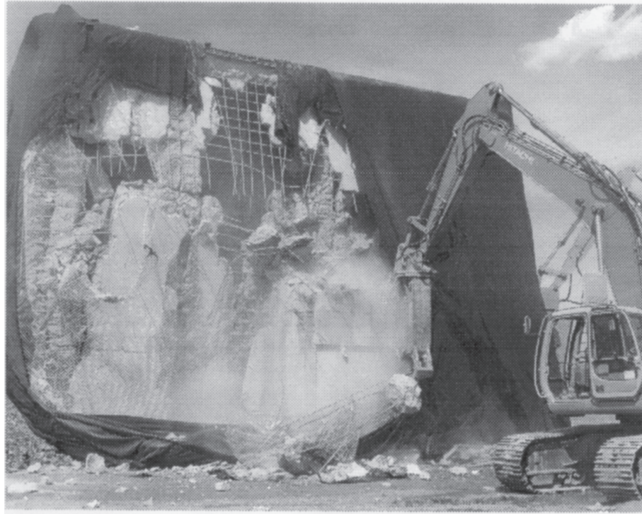
Fig. 89. Walls were easily knocked down on Sunday following the explosive weakening of Saturday, April 13, 2002. Close inspection suggest this was once the south wall because the moveable shield door can just be seen amidst the rubble near the claw of the “processor”.
