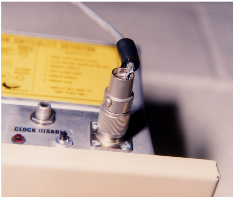
Fig. 133. A broken electronic cable, discovered in September, 1988, was associated with the building's criticality alarm system. The damage was repaired before any consequences occurred; and alarm coverage was never lost.
