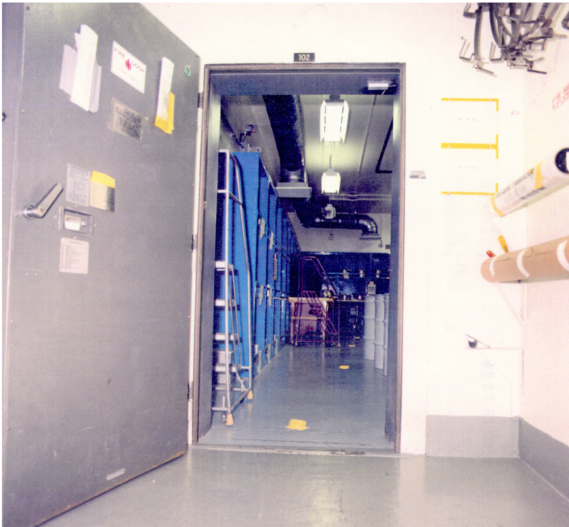
Fig. 38. Room 102 was about doubled in size during the first half of the 1980s; and a bank-vault-like door installed for materials safeguards measures. The shelving was rearranged around the walls of the room for better access to fissile materials. This configuration also left room in the center for waste drums and other equipment.
