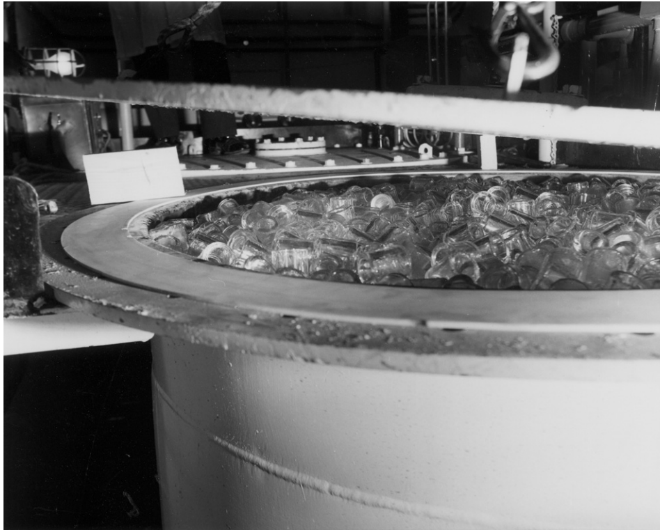
Fig. 116. Raschig rings in the Waste Water Holding Tank (Tank #440) in the Holding Pit as they existed after filling the void discovered April 8, 1976. The void took 1227 rings to fill. The tank's lid is just about to be lowered into place and bolted down.
