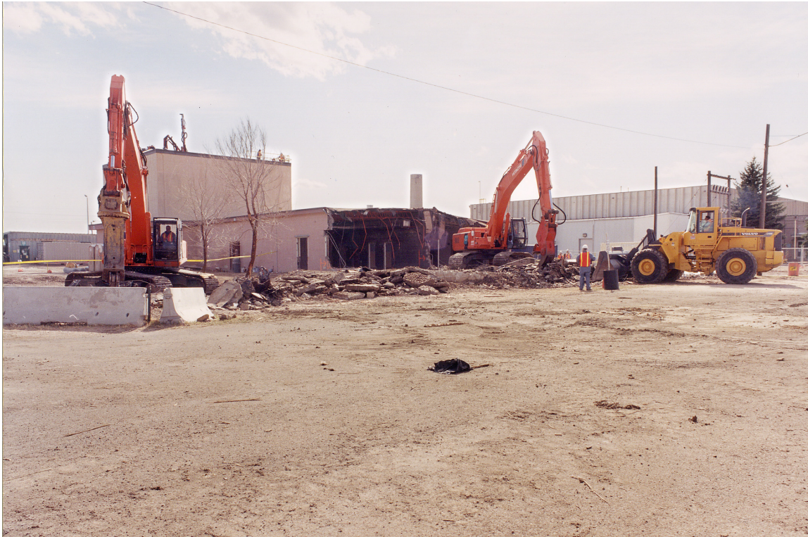
Fig. 84. Heavy demolition equipment had clawed away most of the Office Area by the end of March, 2002. The $175,000 apparatus used to drill holes in walls of the Assembly Room for its eventual explosive fracturing can be seen on the roof.
