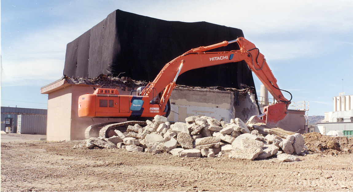
Fig. 86. The Office Area was gone; and only the Assembly Room and the Vault Room remained standing on April 9, 2002. The Assembly Room was later explosively fractured on Saturday, April 13, 2002. It had been covered in chain link fencing to control concrete movement and a layer of black plastic to control dust and debris. The Hitachi tractor was called “the claw” by workers; but management preferred the term “processor.”
