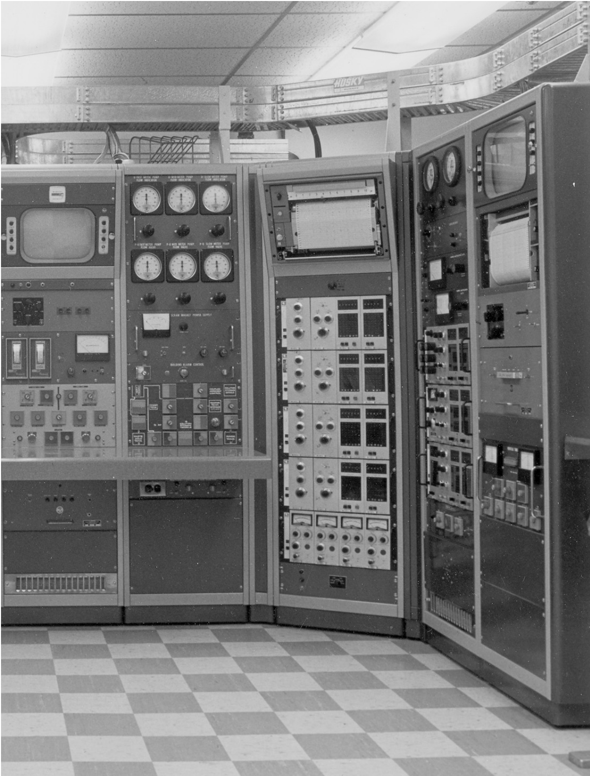
The four individual panels just above the horizontal writing surface controlled “Reactivity Addition Devices.” These and several other functions are described in considerable detail in the text.
